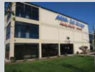
5684 Haden Road Virginia Beach, VA
