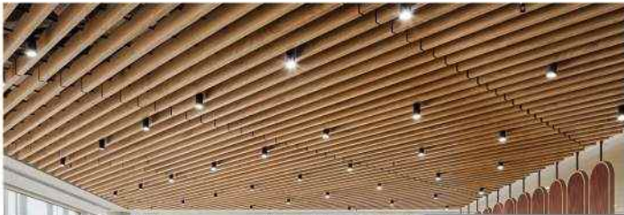
RECEPTION WOOD SLAT CEILING FEATURE
